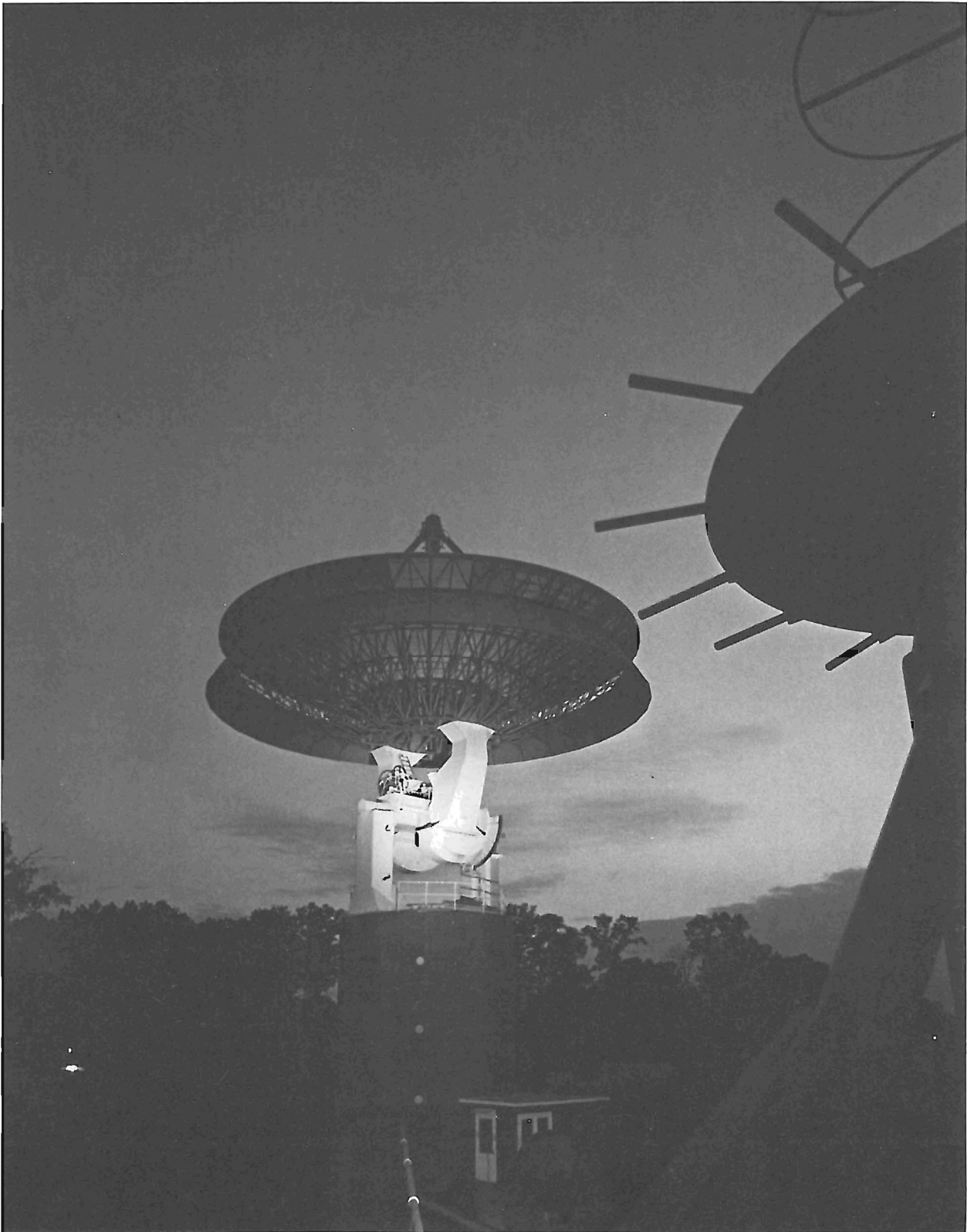
The APL 60-foot-diameter parabolic antenna for transmitting commands to and receiving telemetry from some orbiting satellites.
